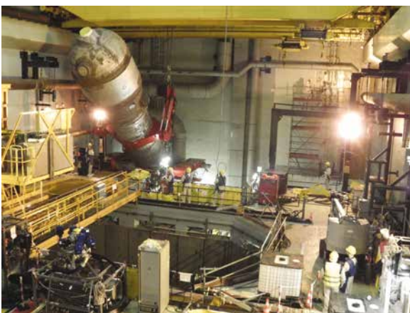
FIGURE 19 - EXTRACTION DES GVS DE CHOOZ A
